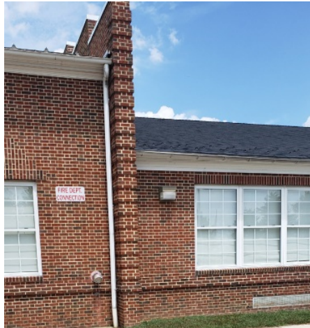
Photo #13 Typical Exterior Wall Pack
