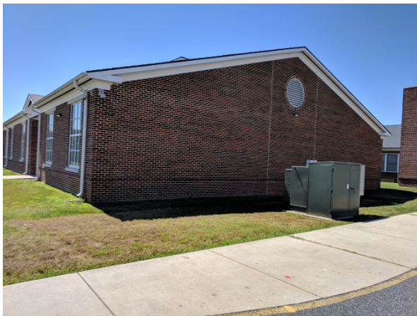
Photo #15 Exterior Lighting on the 2006 Addition
